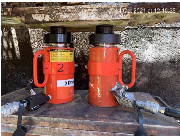
Photo showing two 55 t jacks setup below the cross girder.
