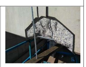
Damaged Deck Units prepped and 6mm stainless steel pins installed to provide a mechanical key.
