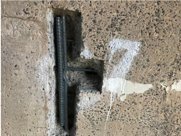
Steel reinforcement replacement
