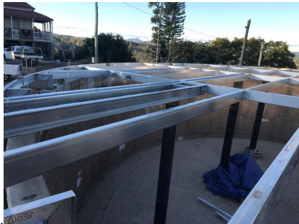
New Aluminium Roof Structure
