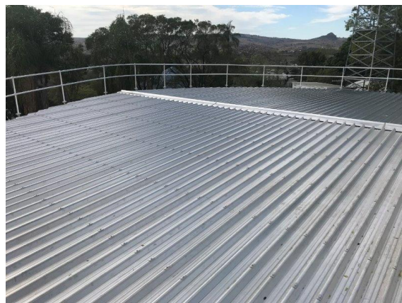
New Aluminium Roof and perimeter handrail
