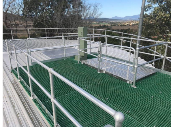
Roof platform and access hatch
