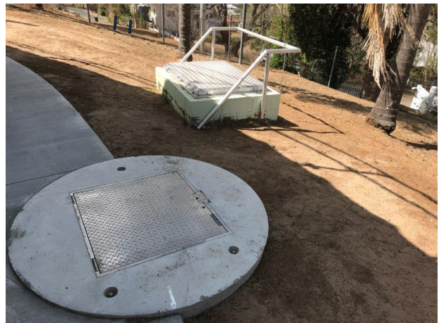
Manhole and flow meter covers
