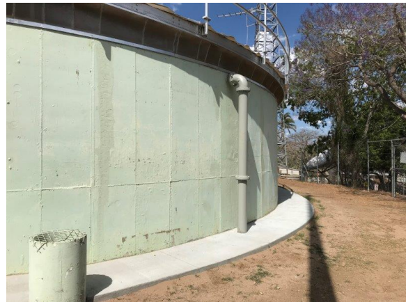
Newly coated overflow pipe and perimeter apron
