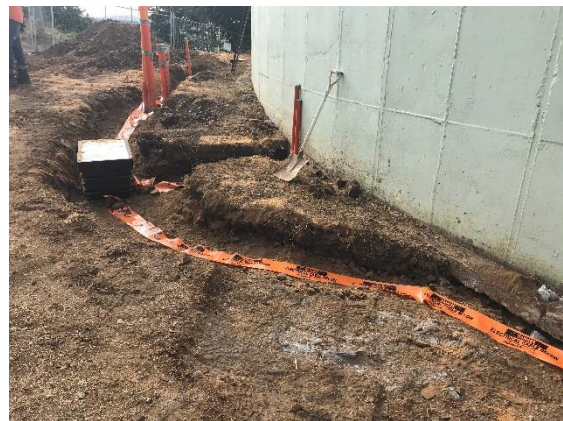
Trenching for electrical ducts and service pits
