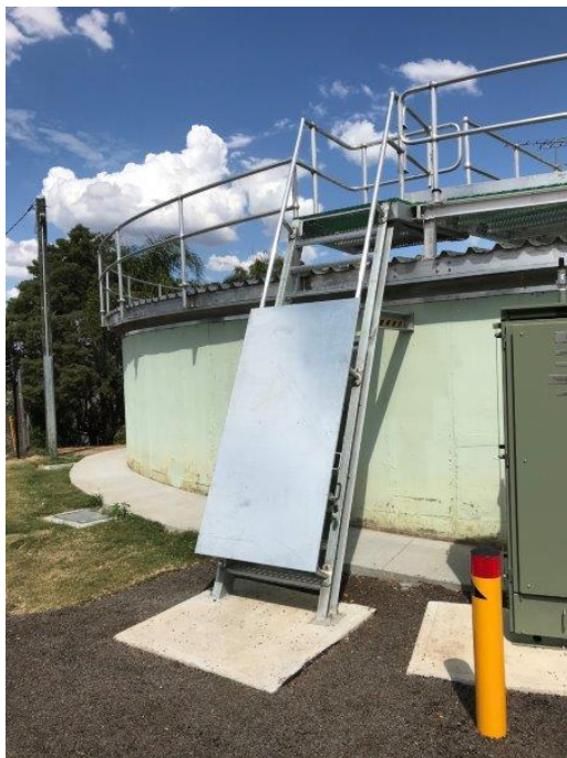
New stepladder with anti-climb security
